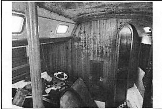
Mold in Cabin
